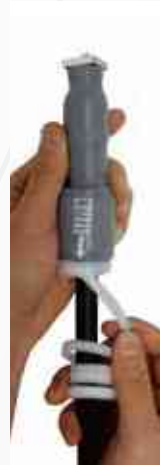
Taking off support core
